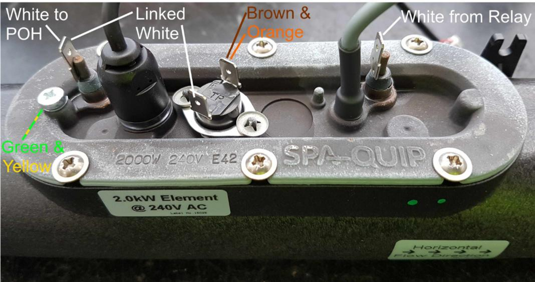
Incoloy Heater Element post Nov 2015 wiring connections
