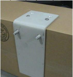
4. Mount the adjustable base to the fixed mounting plate using the pre cut slots, This allows you to adjust the height accordingly. Fasten the adjustable base using the nuts and star washers provided.
