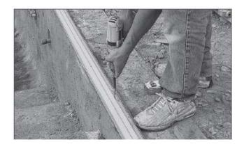
6. The above steps should be carried out down the lengths of the pool only. Any excess track should overhang into the pit. The encapsulation track should overhang into the non pit end by 2" (50.8mm) (see Fig 1.4), this allows for the end pulley to be set into the pool wall (pulleys installed later). <u>At no point should you cut any track.</u> Please ensure that the black plastic protection strip (provided) is used to prevent any concrete falling into the inner guide.
