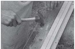
5. Move the encapsulation back over the holes and tighten the screws provided through the encapsulation into the rawl plugs.
