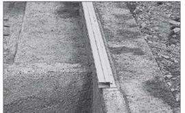
3. Once the encapsulation is set into the correct position, drill though the back flange of the encapsulation approximately 2 <sup>1</sup>/<sub>2</sub>" (63.5mm) deep.
