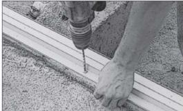
4. Move the encapsulation back a few inches to expose the holes and tap in the rawl plug.
