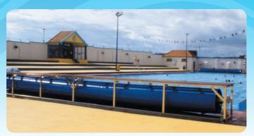
a 152mm (6") or a 304mm (12") diameter stainless steel tube. A 6:1 reduction gearbox is fitted as standard for ease of use, alternatively, this system can be motorised.
